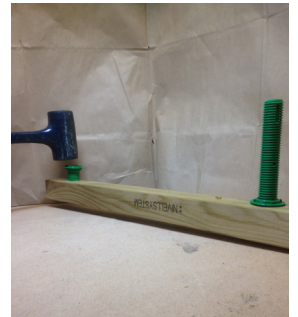
Example of installing a threaded sleeve.
