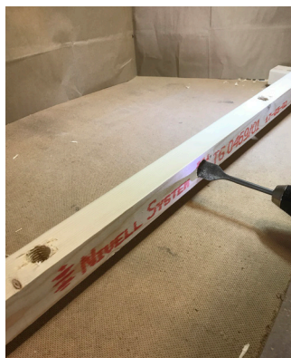
Drilling a transverse hole for installing a threaded sleeve and support against a wall.
