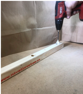
Bore a hole with a 26 mm bit.
