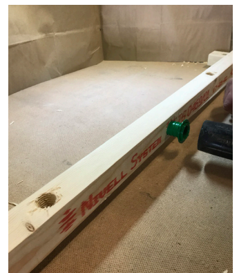
Drilling a transverse hole for installing a threaded sleeve and support against a wall.
