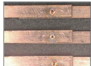
Welding of bus bars
