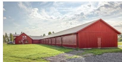
OUR CASE: THE HYDRO66 DATACENTER IN BODEN CHALLENGE: HOW TO COLLECT AND TRANSPORT LOW TEMPERATURE AIR?
