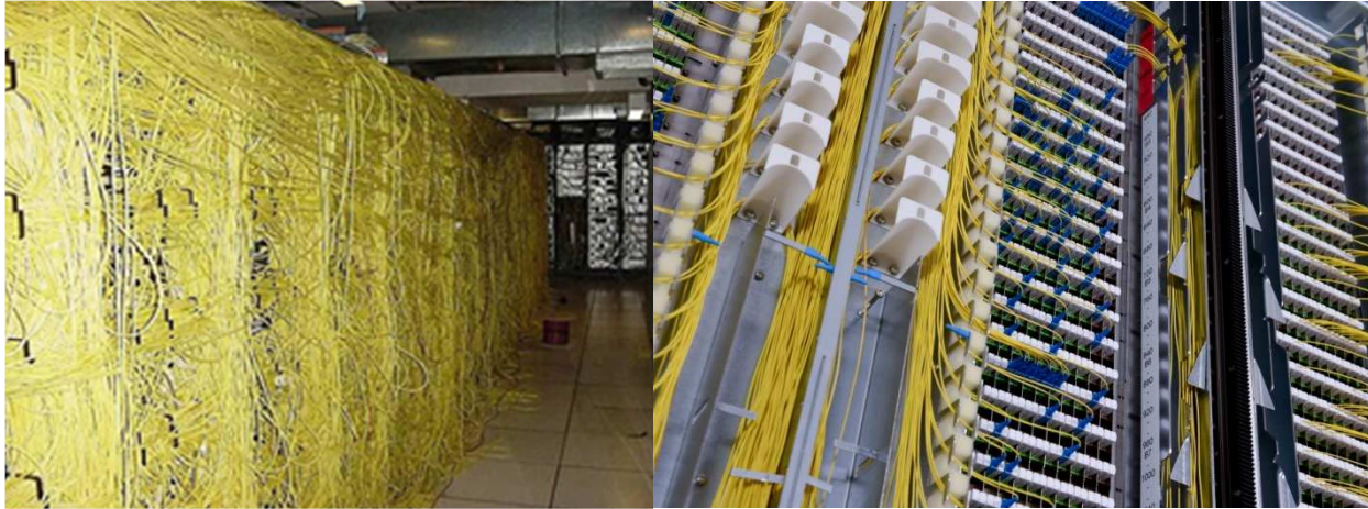
A traditional ODF (left) versus the clean management on an automated panel (right)
